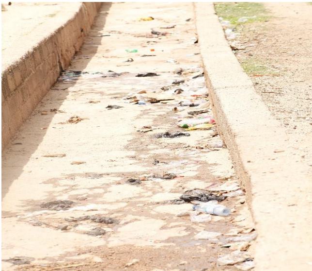
One of the drainages clean by the community members
