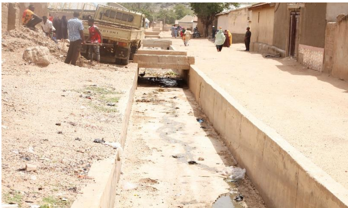
Some youths voluntarily clearing up some drainages in their community.
